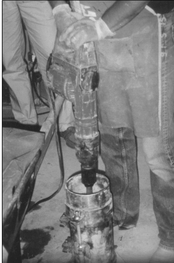
**Figure 4.2**—Preparation of RCC cylinders with a vibrating hammer.
