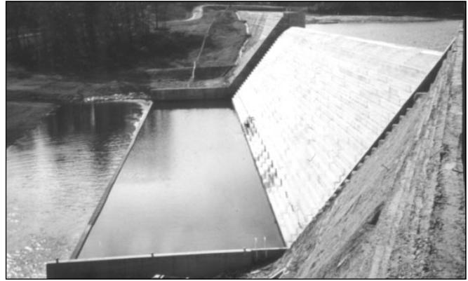
Figure 6.5. Big Haynes Dam, GA, showing training walls to contain and direct flows over the spillway and into the stilling basin.
