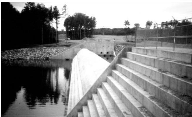
**Figure 6.2. Cast-in-place concrete ogee crest and precast downstream steps for North Tyger River Dam at Spartanburg, SC**
