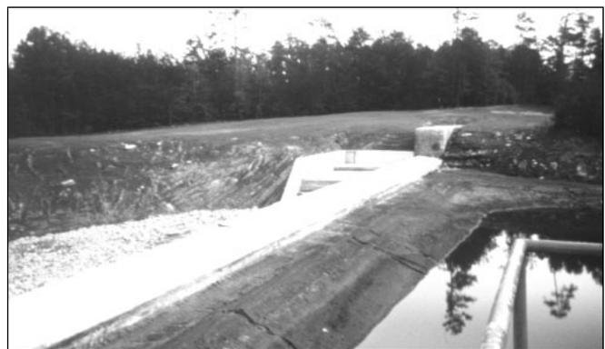
Figure 7.4. Compacted clay berm used to help form and decrease seepage for Tobesofkee Creek Replacement Dam, GA (lake in drawdown condition)
