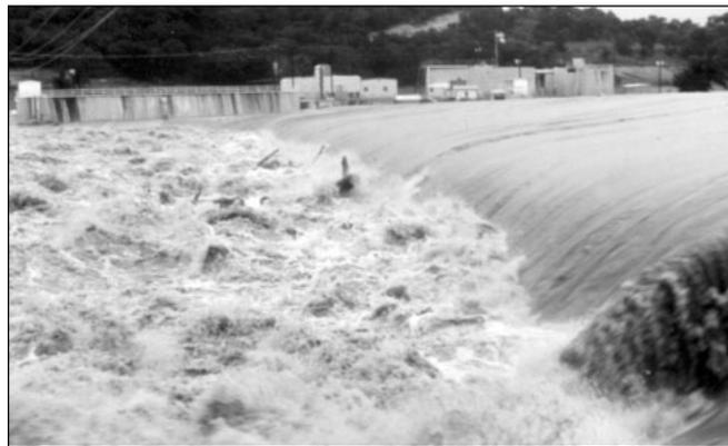
Figure 7.14. Kerrville Ponding Dam, TX being overtopped by 16.2 ft (4.9m) in 1987
