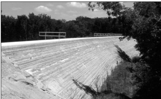
Figure 7.12. Completed stepped downstream face for Woody Branch Detention Dam, TX
