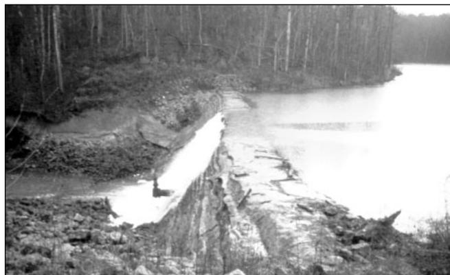
Figure 7.15. Shows operation of RCC spillway for Lake Grace Dam, AL
