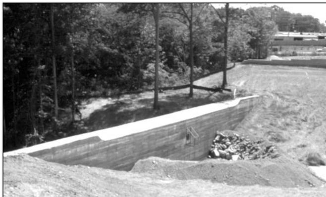
**Figure 7.5 Formed RCC vertical face with some grout-enriched RCC for a portion of Atlanta Road Dam, GA**
