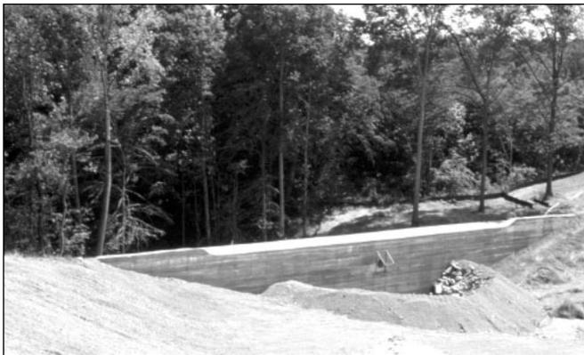
Figure 1.6. Atlanta Road Dam in Georgia stores storm water at a cramped site near Atlanta.
