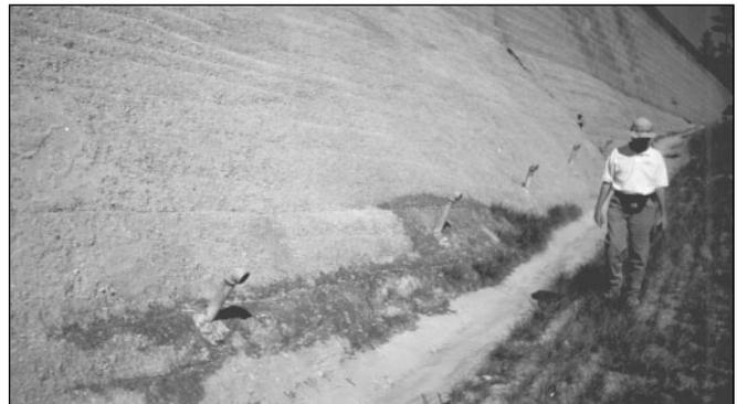
Figure 7.1. Series of steel pipe relief wells along the downstream toe of Big Haynes Dam, GA
