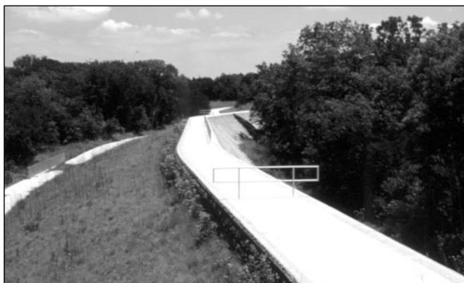
**Figure 7.6. Grassed earth berm on upstream face of Woody Branch Detention Dam, TX**
