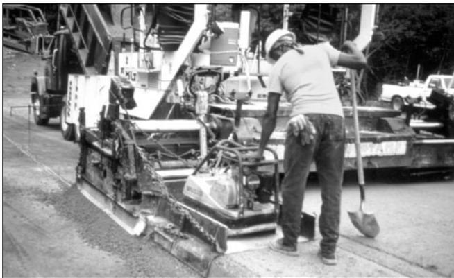
Figure 7.11. Slip-form attached to tamping paver used to form 1-ft (0.3m) high steps for Woody Branch Detention Dam, TX
