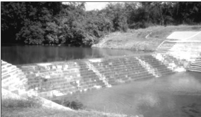
Figure 1.2. North Bosque River Channel Dam diverts water for the Clifton, TX water supply system.
