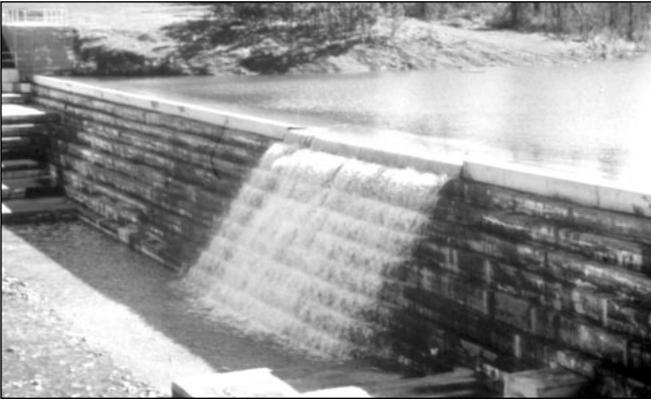
**Figure 7.16.** Two-foot (0.6m) high steps of formed RCC for Tobesofkee Creek Replacement Dam, GA provide hydraulically efficient and visually attractive spillway
