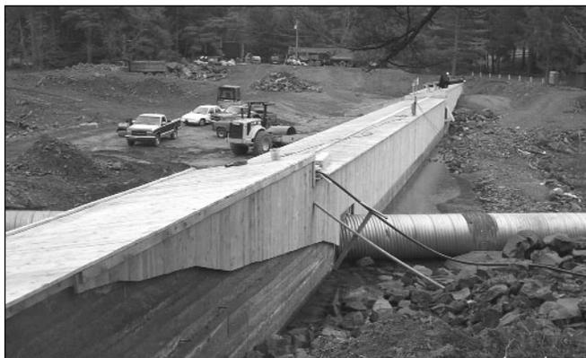
Figure 1.8. Rebuilt Bear Creek showing timber planks being installed along downstream vertical face of new RCC dam.
