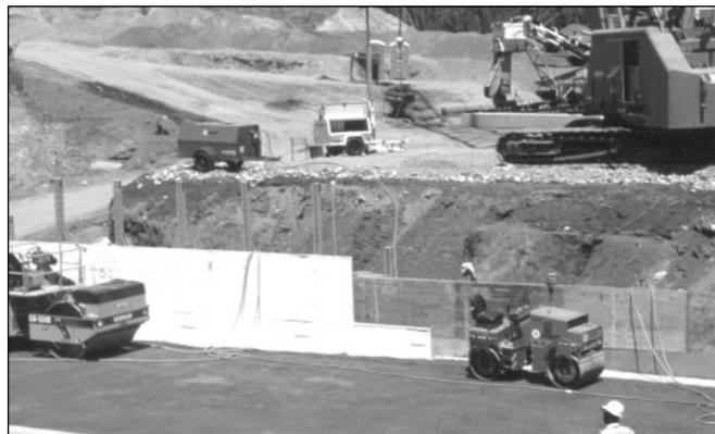
**Figure 7.7. Membrane-faced precast concrete panels form upstream vertical face of North Tyger River, SC water storage dam**
