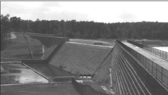
**Figure 3.3. Big Haynes Dam near Conyers, GA built in monoliths with a break in the axis.**
