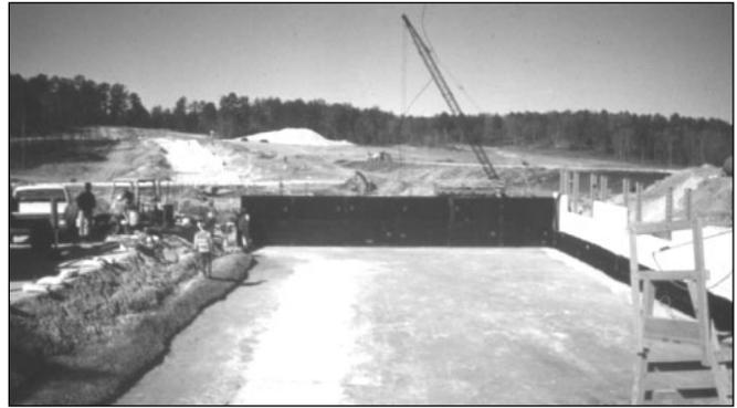
**Figure 3.4. Prepared soil foundation for Big Haynes Dam, GA. Note trench drain.**
