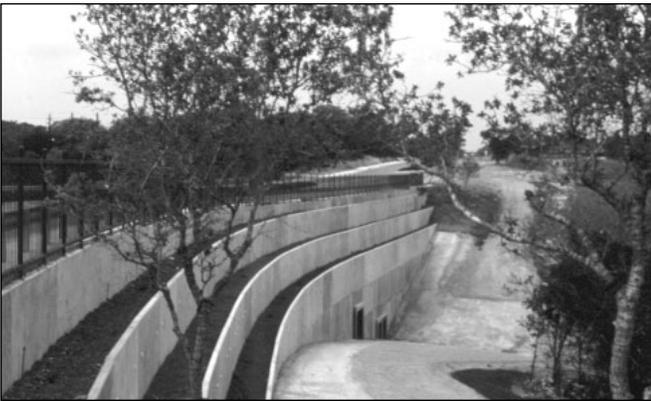
**Figure 7.17.** Precast panels to form downstream planter boxes for North Loop Detention Dam No. 1, TX
