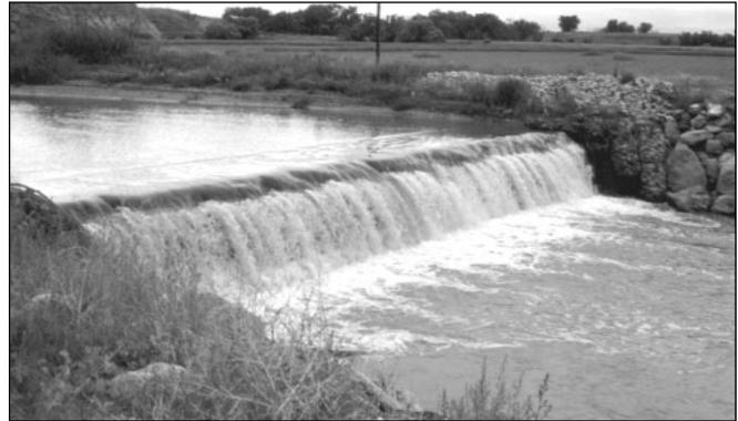
**Figure 1.4.** Sahara Diversion Ditch Dam near Kaycee, WY diverts water for irrigation.
