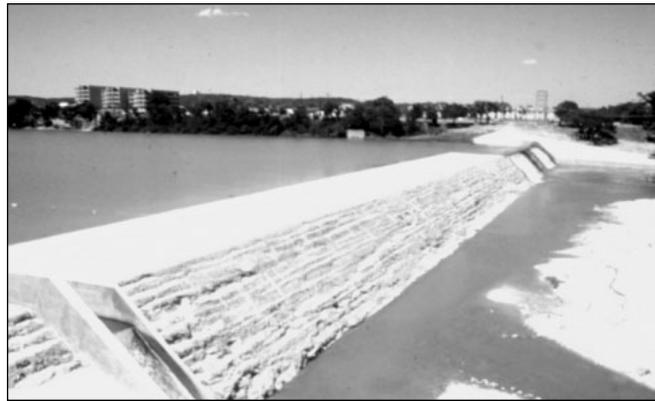
Figure 7.13. Uncompacted RCC downstream face for Kerrville Ponding Dam, TX following overtopping
