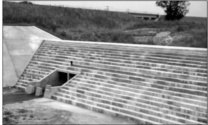
Figure 7.3. Formed RCC steps for Prairie Creek Detention Dam, TX
