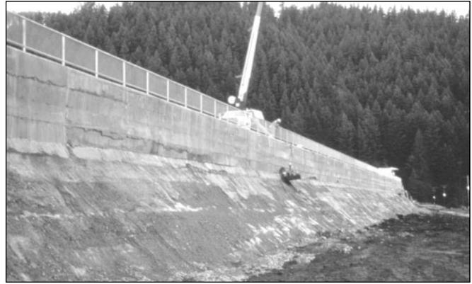
**Figure 7.18.** Partial replacement for Faraday Dam, OR has vertical formed chimney section plus unformed RCC downstream
