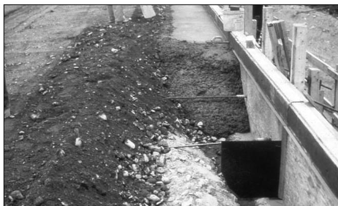
**Figure 7.8. Monksville Dam, NJ, shows where RCC was placed first followed by conventional concrete to form upstream vertical face**
