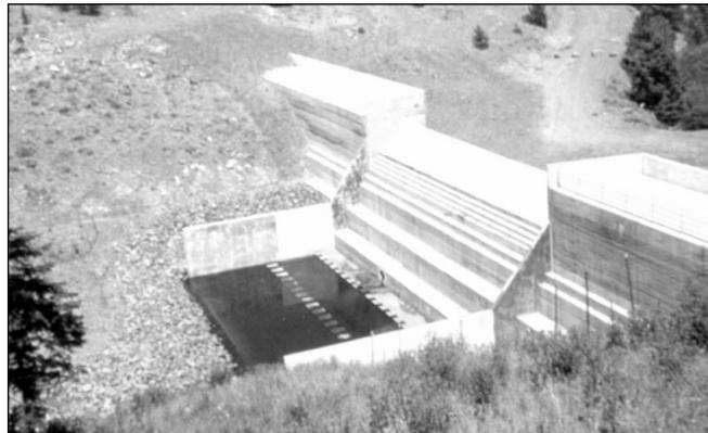
Figure 7.19. Completed Bullard Creek Dam, OR which includes exposed RCC steps
