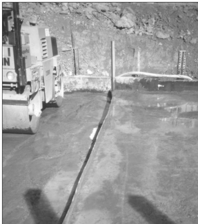
Figure 7.20. Contraction joints consisting of galvanized metal sheets
