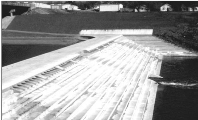
**Figure 6.4. Broad crested weir and series of corrugated metal conduits at the crest of the 4th Street Low Water Dam at Ft. Worth, TX**
