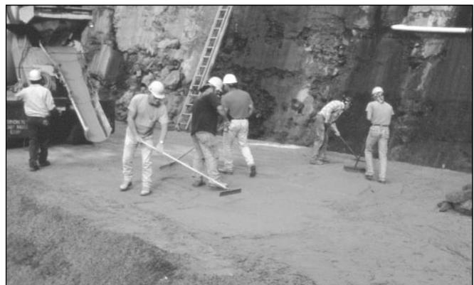
Figure 7.21. Spreading bedding mortar from a transit-mixed concrete truck with brooms
