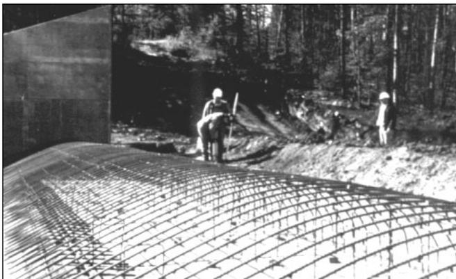
**Figure 6.1. Ogee crest being constructed for Tellico Saddle Dam, TN**
