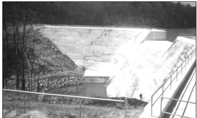
Figure 6.6. Hudson River Dam No. 11, GA, showing spillway with no training walls.
