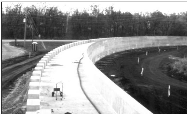
**Figure 6.3. Sharpened crested weir and concrete energy dissipation blocks at the crest of Whipps Mill Dam at Louisville , KY**
