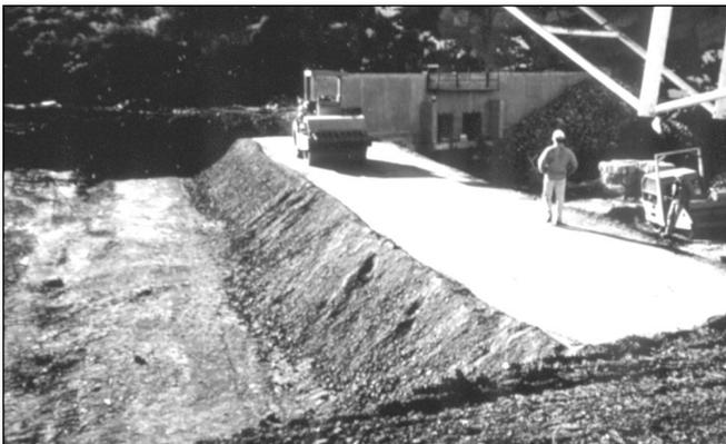
Figure 7.2. Unformed RCC face for Sahara Ditch Creek Diversion Dam, WY.
