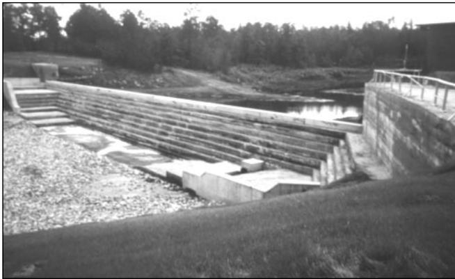
Figure 7.10 . Two-foot (0.6m) high exposed RCC steps for downstream face of Tobesofkee Creek Replacement Dam,
