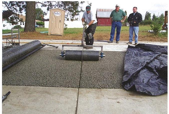
Figure 14. Joint roller, commonly referred to as a “pizza cutter.” (R. Banka)
