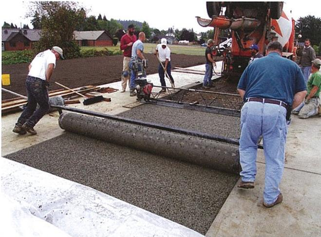
Figure 13. Compaction of pervious concrete with a steel roller. (R. Banka)
