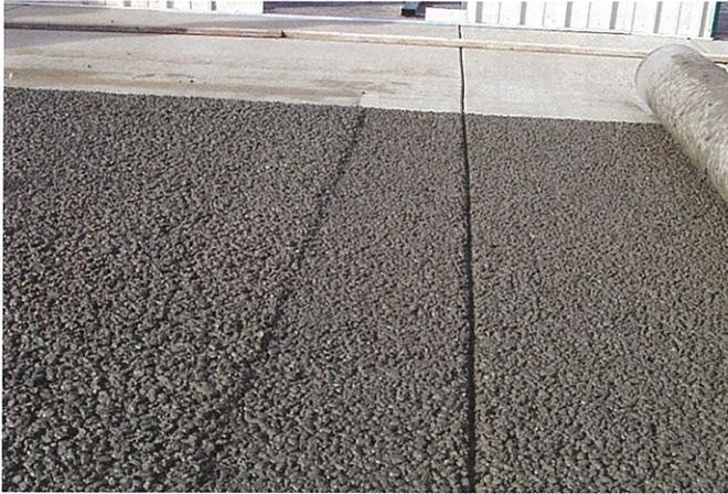
Figure 12. Pervious concrete after screeding (left) and after compaction (right). Note the joint aligned with previously placed slab to avoid reflective cracking. Roller used for compaction is visible on the far right. (R. Banka)
