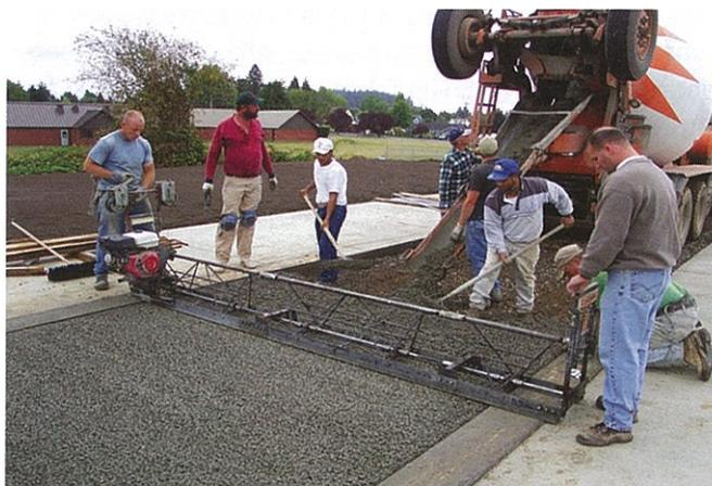
*Figure 11. Pervious concrete is usually placed and then struck off with a vibratory screed. (R. Banka)*
