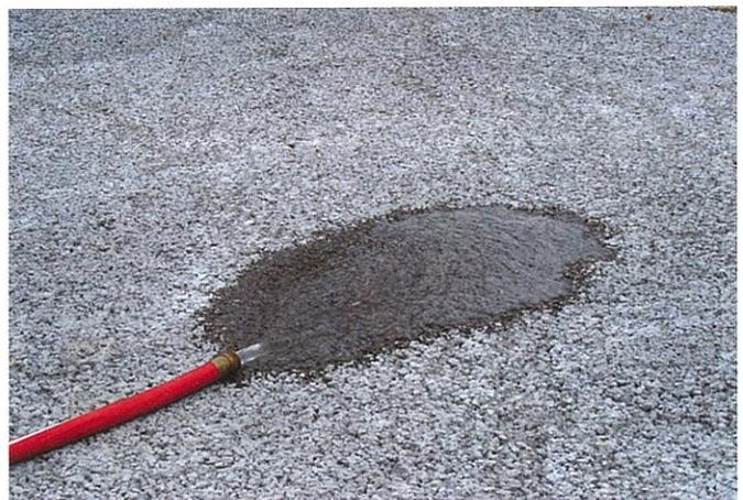
*Figure 1. Pervious concrete's key characteristic is its open pore structure that allows high rates of water transmission. Trail in Athens Regional Park in Athens, TN, (A. Sparkman).*
