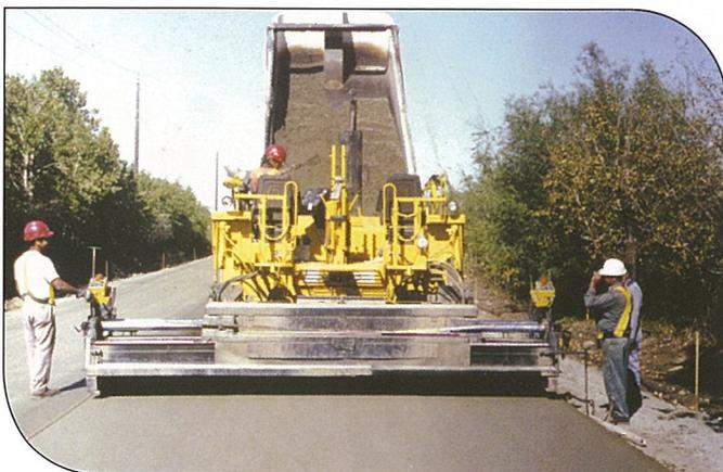
**Road widening made easy with roller-compacted concrete.**
