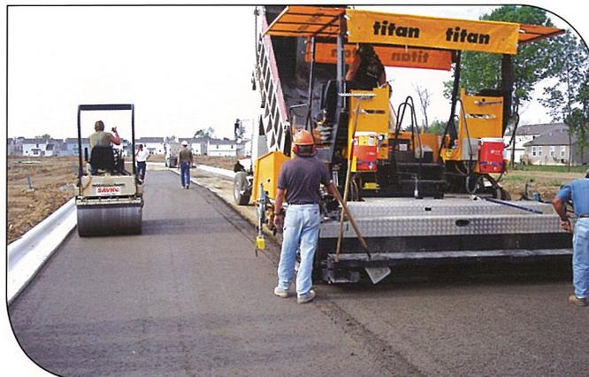
**Constructing city streets in Columbus, OH using RCC is quick and convenient. Residents can drive on the RCC base soon after final rolling.**
