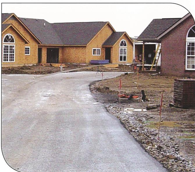
**RCC placed during site work serves as a working surface. With a thin overlay, it becomes a residential street once construction is complete.**
