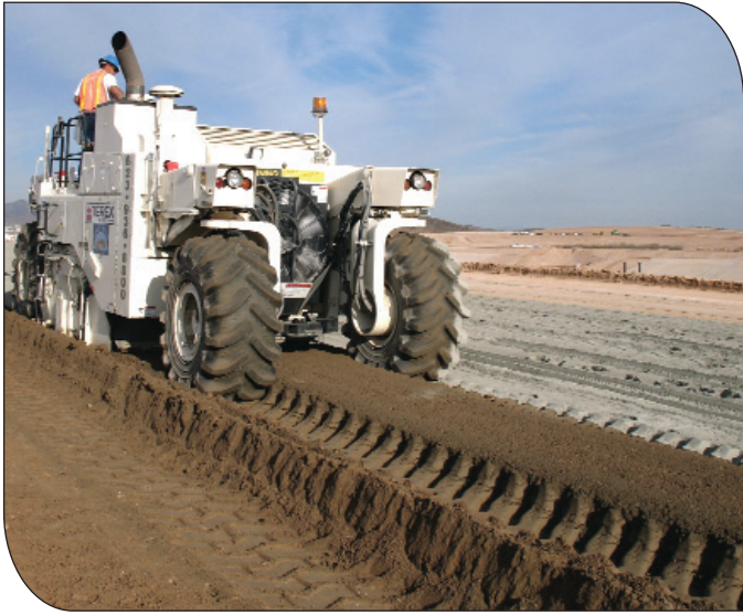
A pulverizer mixing soil-cement.
