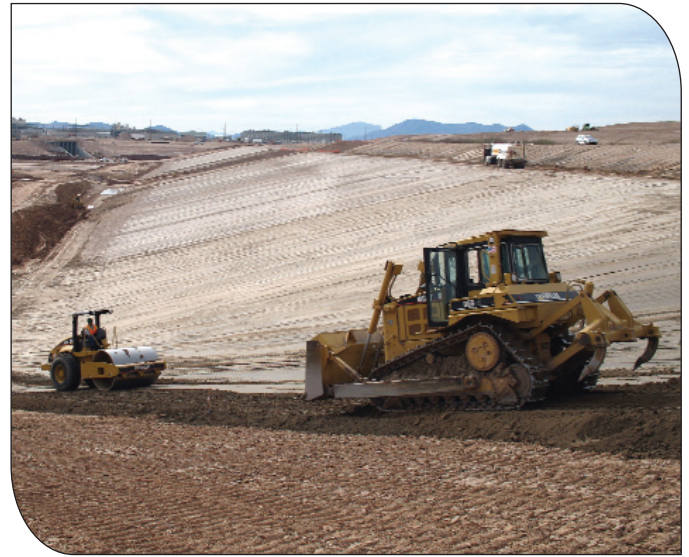
Spreading and compacting soil cement.
