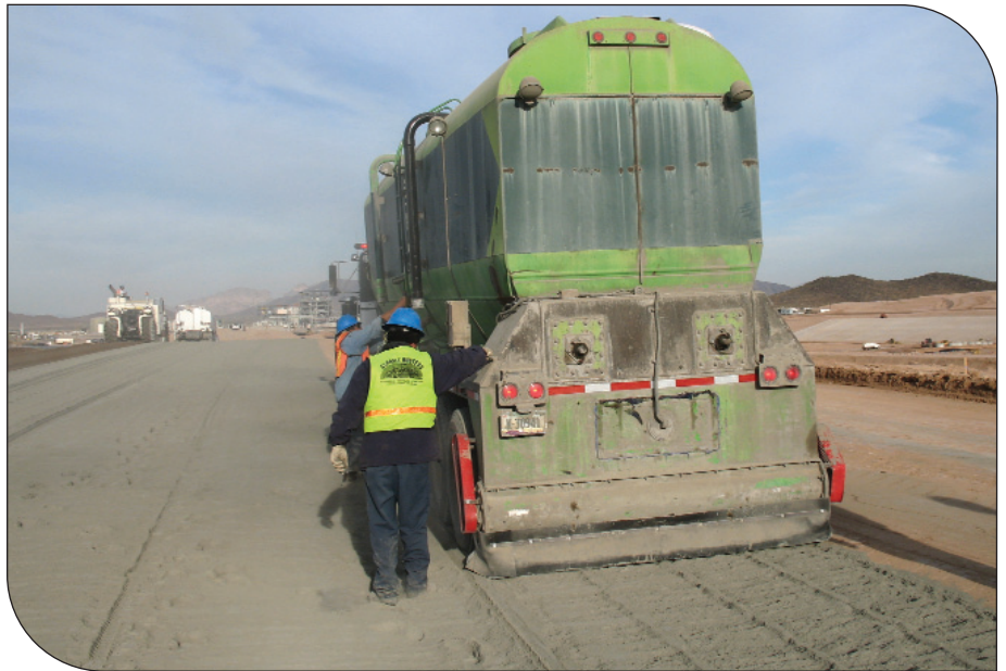
Spreading cement.
