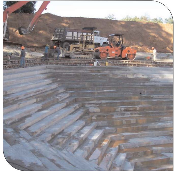
Close-up view of RCC steps
