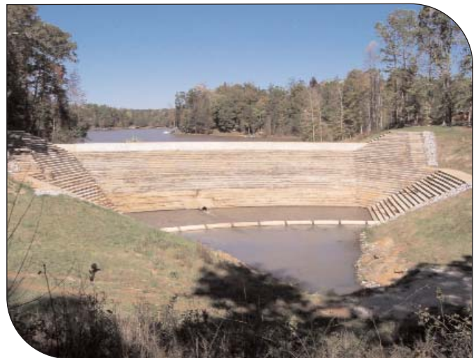
Completed RCC structure
