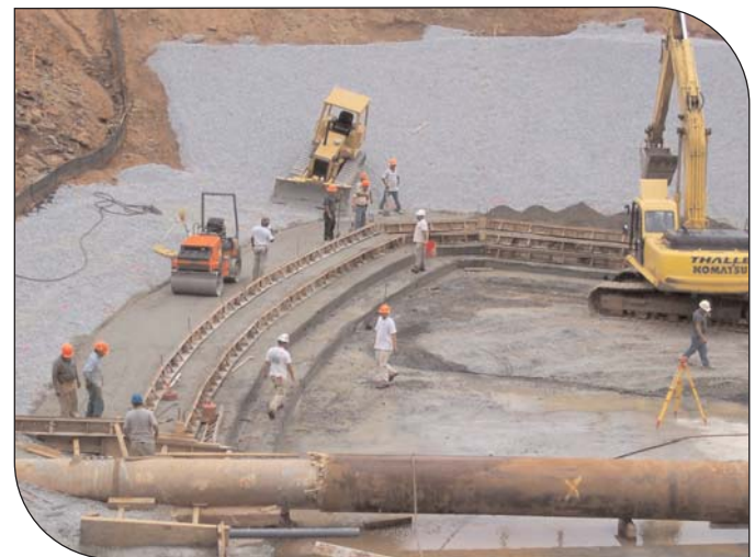
Construction of spillway chute steps and stilling basin training walls
