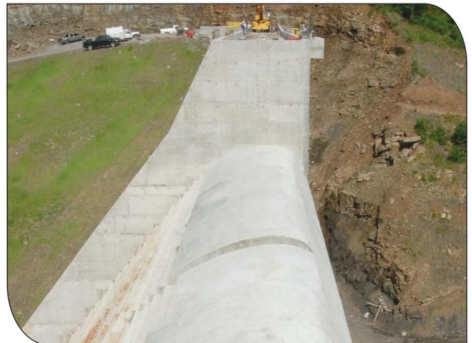
**Uncontrolled overflow spillway looking toward right abutment**
