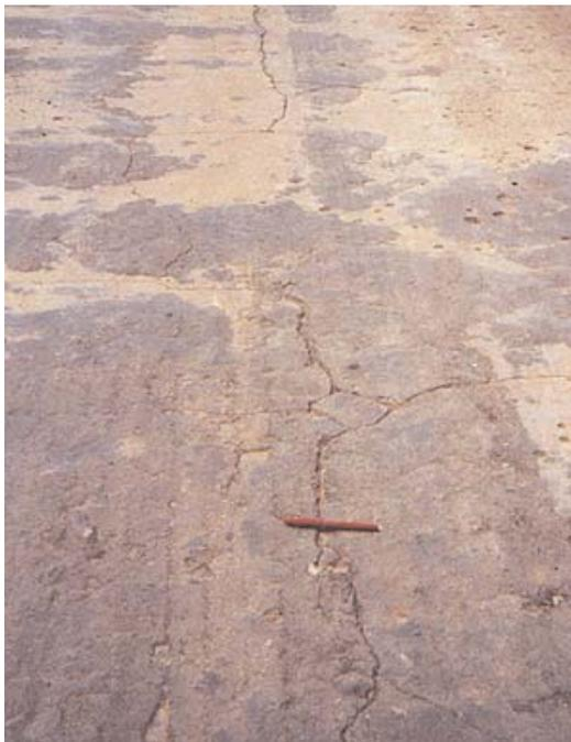
**Figure 3-3.** Longitudinal crack in a 2-week old soil-cement layer.
