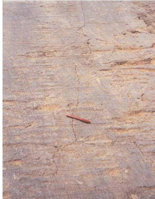
**Figure 3-4.** Cracks in a five-day old soil-cement layer.
