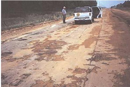
**Figure 3-2.** Surface scabbing resulting from reworking followed by prolonged exposure.
