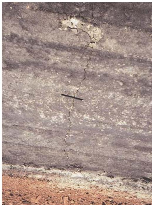
**Figure 3-1. Transverse crack in a 6-month-old soil-cement layer with curing seal.**
