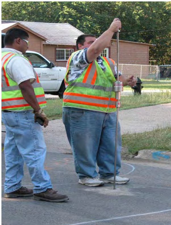
Figure 36. DCP testing device.
