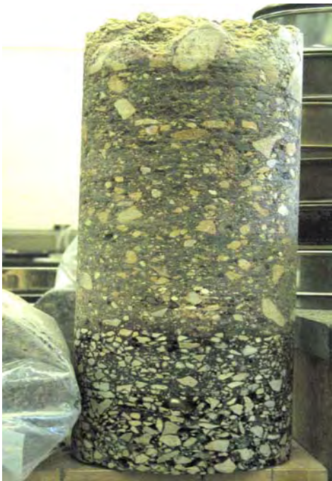
Figure 28. Core from the test pavement after 3 years in service.
