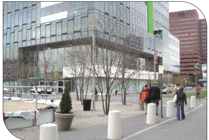
The Genzyme Building at Kendall Square
