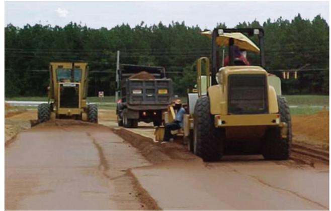
**Figure 3.5.** Soil/aggregate spreading operation working in staggered position across roadway to minimize longitudinal cold joints.
