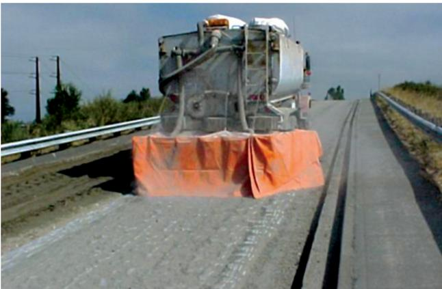
*Figure 3.2. In mixed-in-place construction, cement is uniformly distributed over the area to be processed.*
