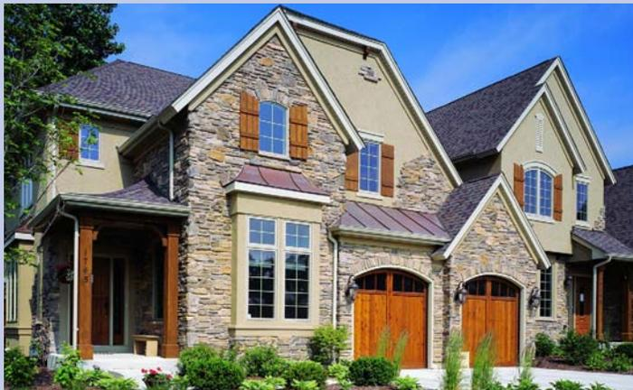
*Fig. 6. Fire safety: the façade of this residence combines two noncombustible finishes, portland cement plaster (stucco) and manufactured stone veneer products, for an attractive appearance. These products are frequently made with white cement.*
