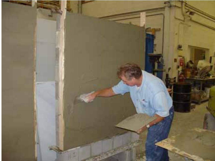
Figure 6— The final step in the building of the walls - the application of the stucco to the block.
