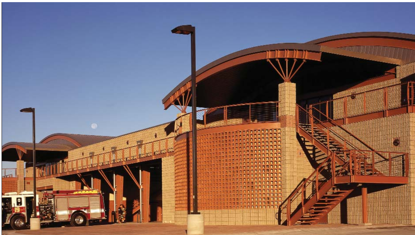
Air Rescue and Fire Fighting Station at Phoenix Sky Harbor Int'l Airport. Photo: Courtesy of National Concrete Masonry Association (For complete photo description, see online material).
