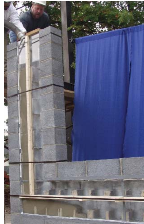
Self-consolidating grout (SCG) moves freely in tight spaces, as seen through the clear plastic face on this demonstration panel.
